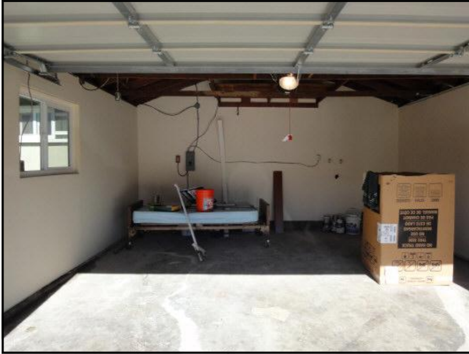
Subject Garage Interior 18487 Del Bonita Street
