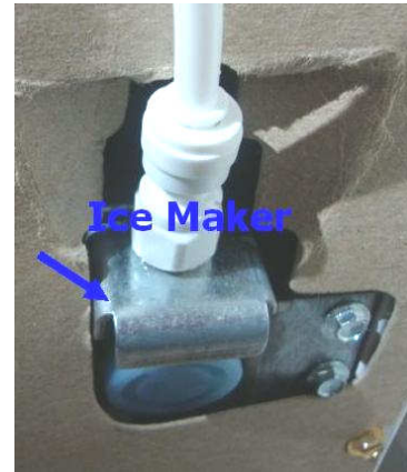
Just screw on the fitting and complete
