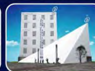
Broad Air-conditioning Pavilion
